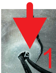
Pass wires from light box into cabinet
