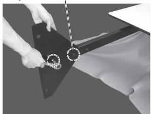
1 There is an L and an R foot frame. Be careful with the direction of the frames. Attach the foot frame to the foot frame bracket. 1 person should support the foot frame and insert the protruding part of the screw holes on the foot frame into the holes on the foot frame bracket, while the other person lightly fastens it in place with 3 hexagon bolts.
